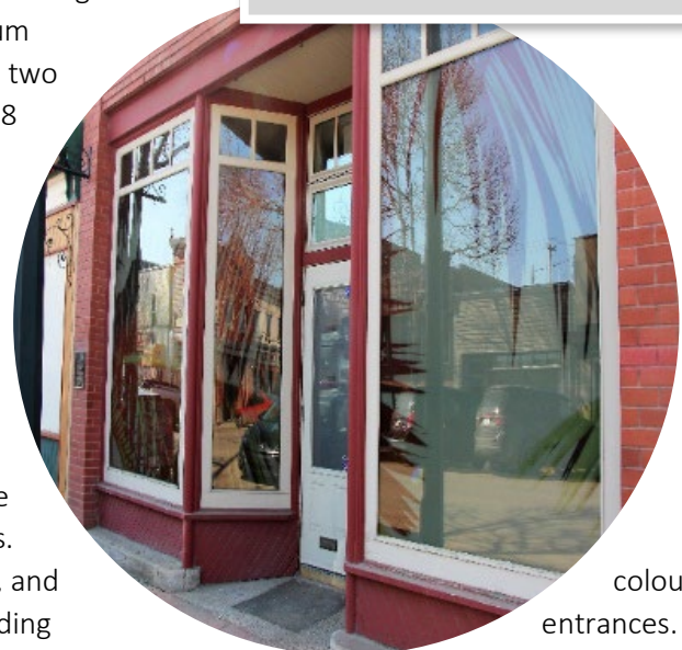
Recessed building entranceway
